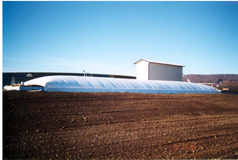
Figure 2-1 A dairy farm anaerobic digestion system (RCM, Inc., Berkeley, California)
