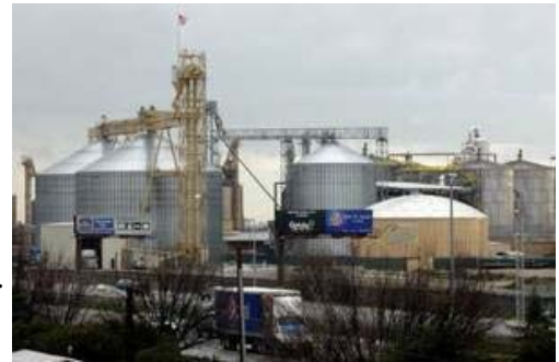
The Cilino ethanol plant, just north and west of Highway 99 and the Keyes overpass, will be leasing to AE Biofuels within the next few months to apparently begin production of ethanol. January 19, 2010 (BART AH YOU/bahyou@modbee.com) --
