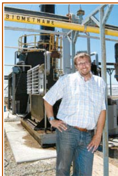
Fresno County dairy farmer David Albers stands next to equipment on his farm that upgrades methane gas from manure produced by his cows into a usable form of natural gas that is piped directly to Pacific Gas & Electric Co. His dairy is the first in the state to deliver pipeline-quality, renewable natural gas to the utility.
