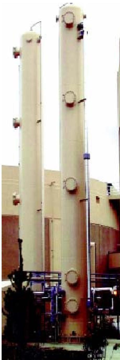
Figure 3-1 Carbon dioxide absorption towers at the King County South Wastewater Treatment Plant
